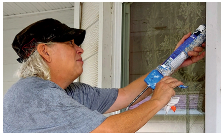
Above | Project Flo volunteer caulks window.
