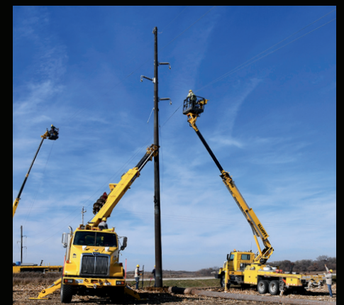
Above | Corn Belt Power transmission crews set new poles along the new stretch of line between Humboldt and Weaver Switching Stations, Nov 2. A little over 14 miles of new transmission line is set for construction.
