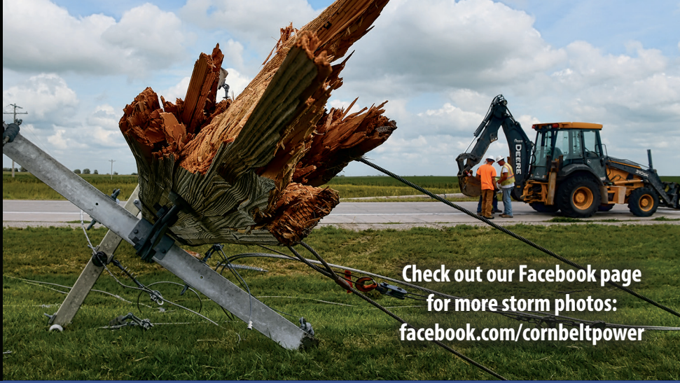
Above | A shattered, laminate transmission pole rests de-energized in the ditch two and a half miles south of Huxley after the Aug. 10 derecho downed this two-mile section of line amongst many others around the state.
